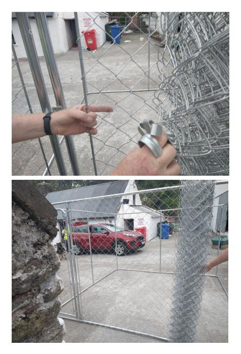
9: Using the wire provided, start securing the wire to the frame. Around the bottom you should tie every 3 chain links and every 4 or 5 at the top and on the uprights.
